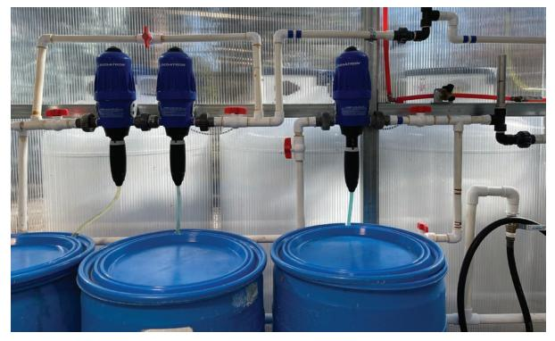
Figure 1. Two Dosatron setups with bypass lines and water hammer arrestors. The left pair supplies a standard A + B hydroponic fertilizer regime, while the single injector to the right supplies a standard 13-2-13 regime for container crops.
